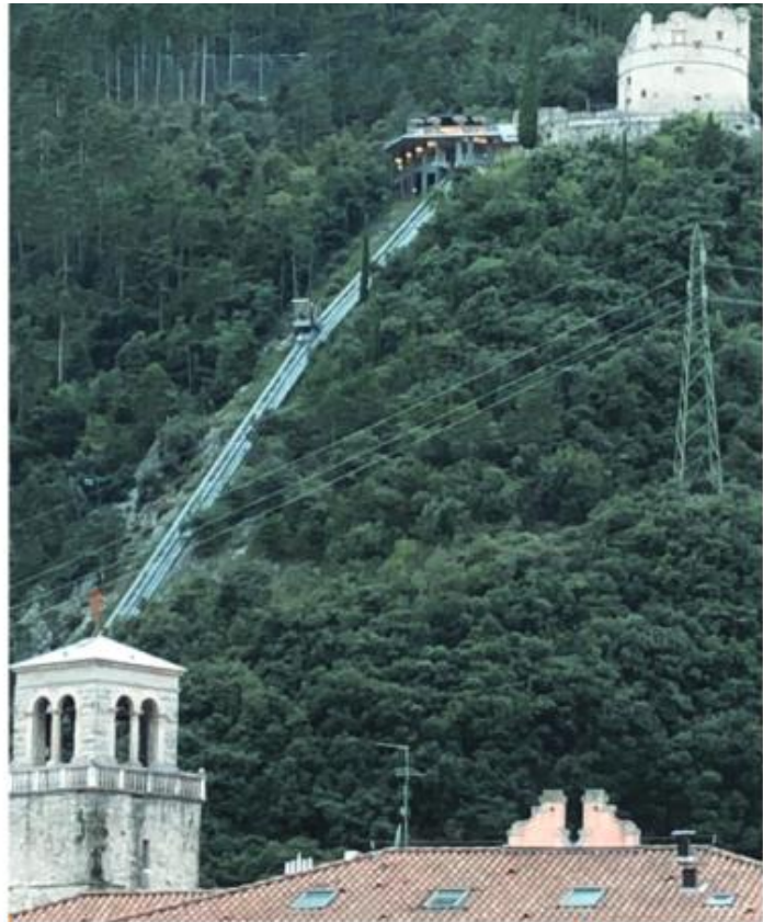
The 208-m track has two stops and can be covered in about 2 min.
