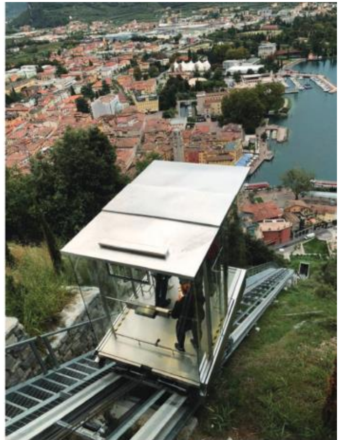
The lift has variable inclination from 37° to 43°.
